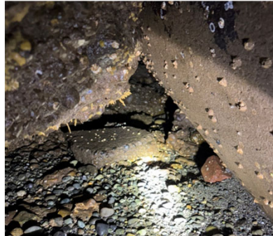
Right: Gap underneath outfall pipe at seawall from south side
